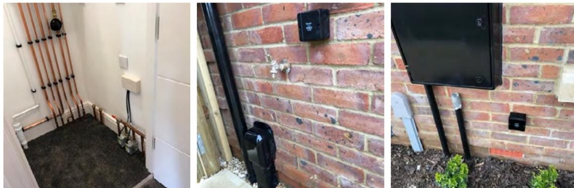
Photos from left to right: 1, Future hot water tank storage cupboard with capped off flow and return ready for future ASHP installation. 2, External capped flow and return with terminated electrical connection. 3, Terminated connection for EV charging connection and electrical duct.
